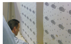
Butt joint treatment with ARDEX ENDURA WPM DECKWEB sandwiched between 2 coats of ARDEX ENDURA WPM 002 No overlap
