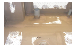
Installation of WPM 1000 X with ARDEX ENDURA GOLD STAR / WHITE STAR / DIAMOND STAR / PLATINUM STAR
