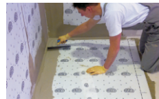
ARDEX ENDURA WPM DECKWEB sandwiched between ARDEX ENDURA WPM 002 in corners
